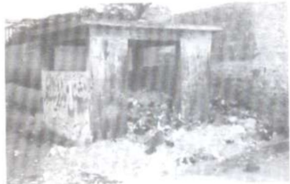
Improperly located and badly constructed garbage collection points.
